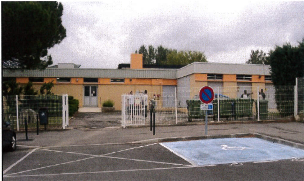
PHOTO 1 – FACADE NORD - ENTREE DE SERVICE
